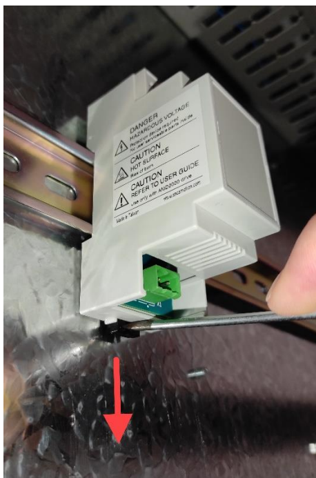
Figure 6-13 Unmounting the Soft Start Module from the DIN rail
