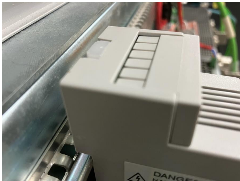
Figure 6-12 Ensure the white DIN rail clip is fully inserted
